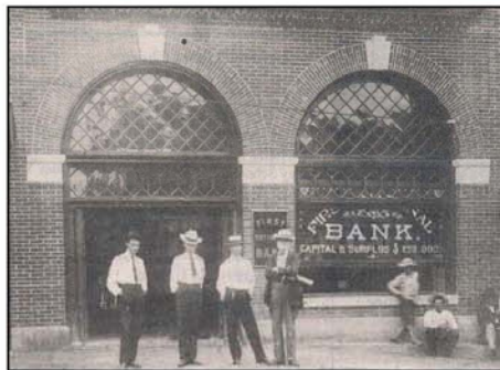
Historic view of First Bank of Farmersville
