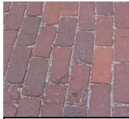
The brick streets are original, and date to the 1920s.
